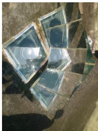
Figure 10: Accumulation of moisture
