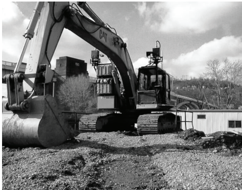
Figure 6. Autonomous excavator with sensors mounted for unmanned operation
